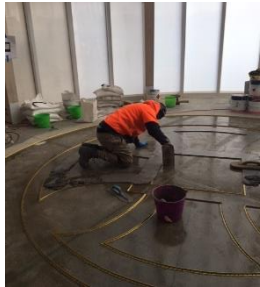
Installation of Brass Strip
