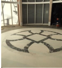
Architectural Terrazzite has been installed
