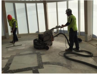
Grinding Process underway
